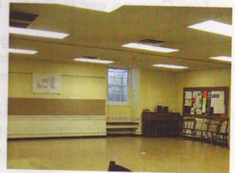
Assembly room ceiling
