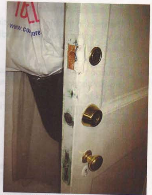
Door at office (112)
