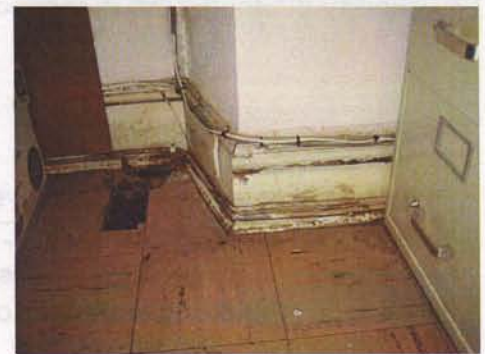
Baseboard at office (108)
