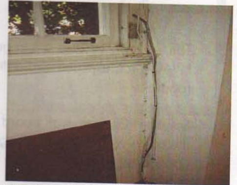
Window at office (108)
