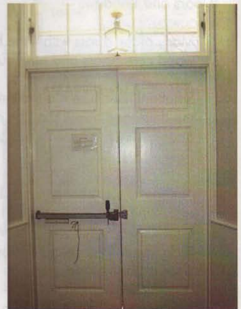
Second floor vestibule doors in hall
