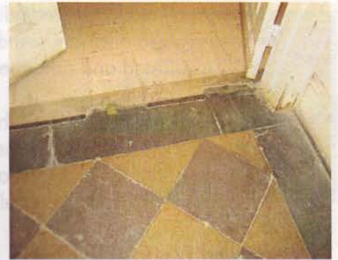
Original tile at storage room (102)
