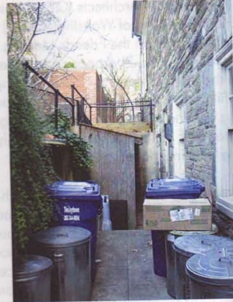
Areaway at Kitchen
