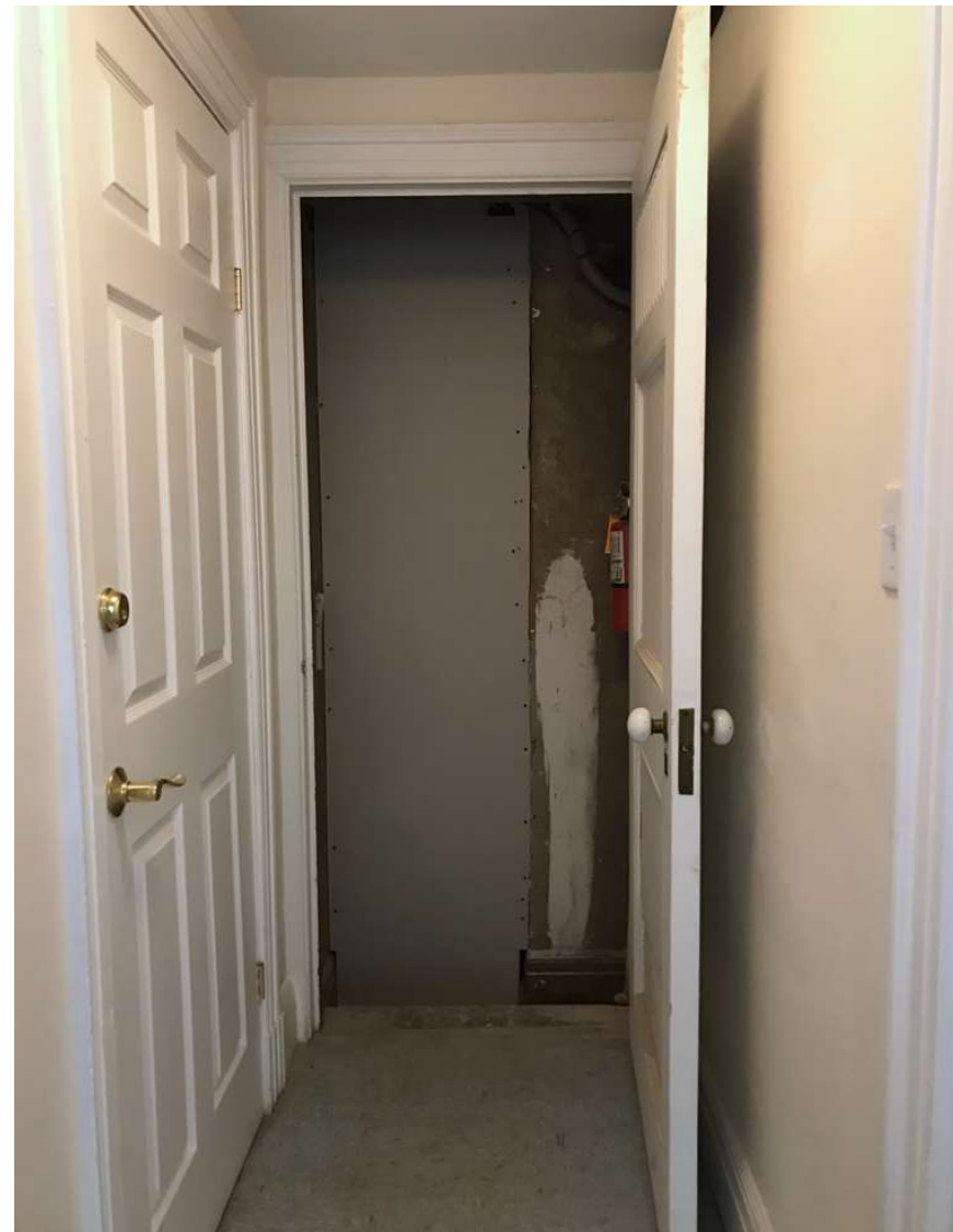
A wall has been added to the janitor's closet (formerly Quaker House Boiler Room). We hope the carpenter remembered to step outside before adding the wall, as the room now has zero doors.
