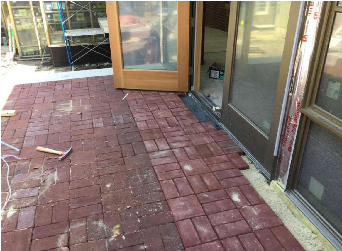
A pair of masons extend the Quaker House patio brickwork.
