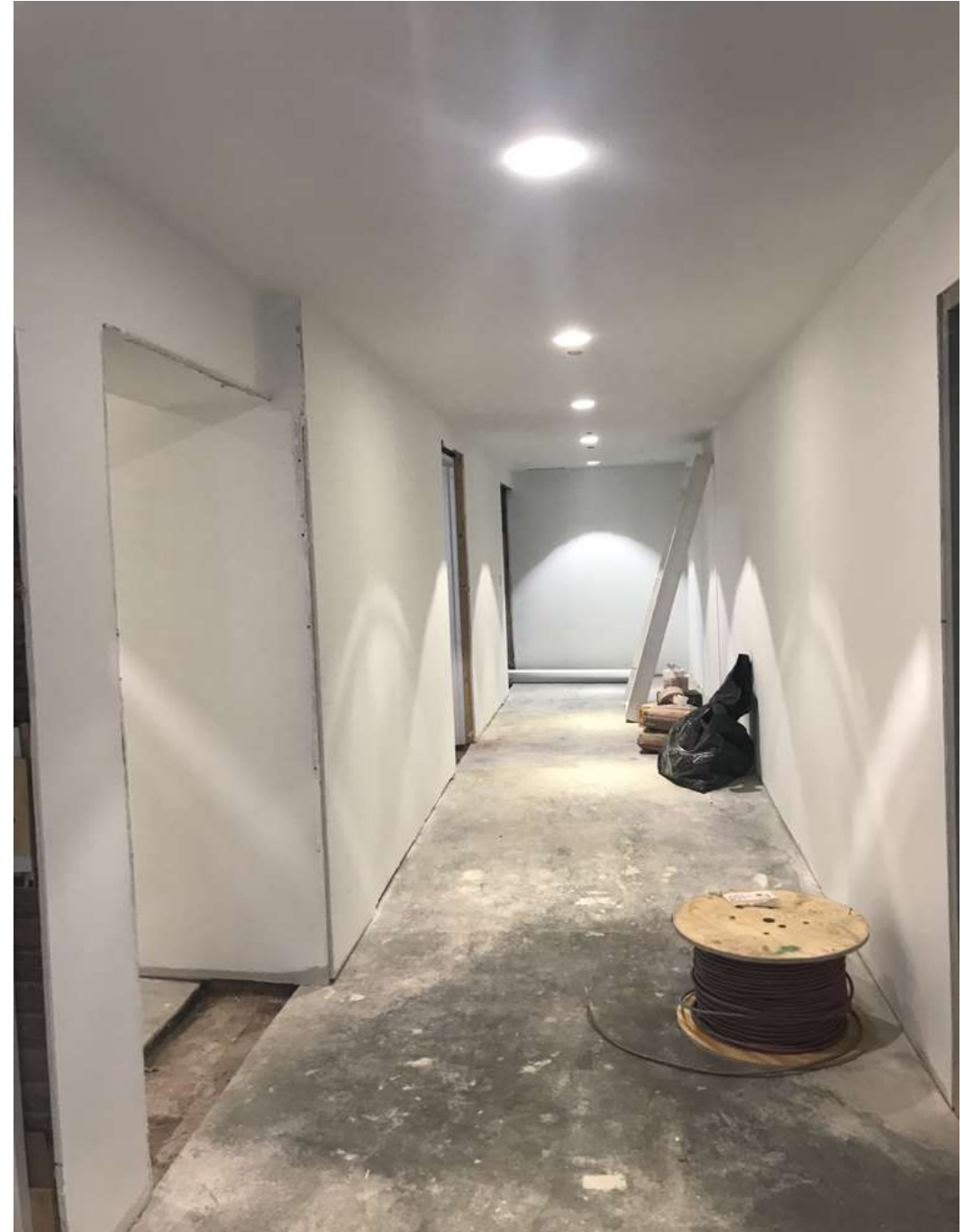
One painter primes the ground floor rooms and hallway.
