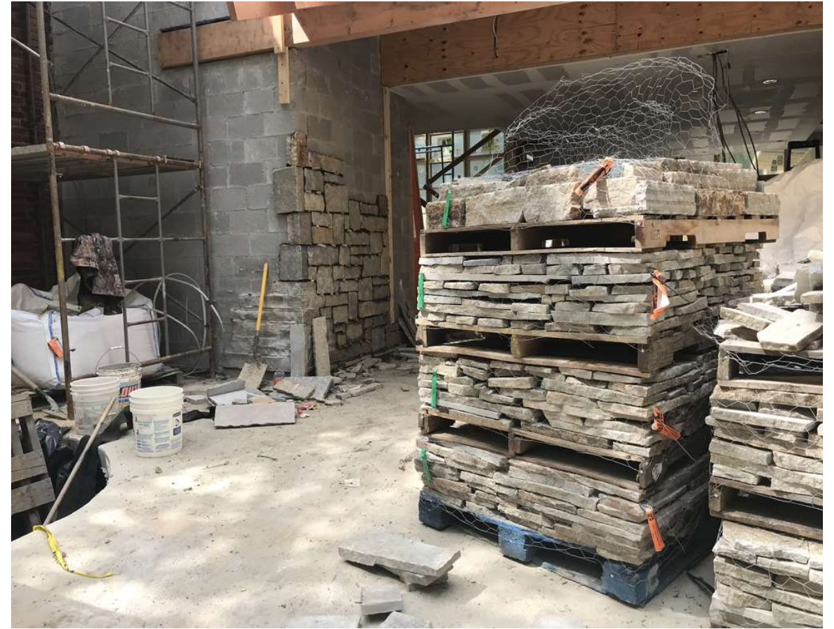
One mason starts to lay up stone on the elevator shaft.
