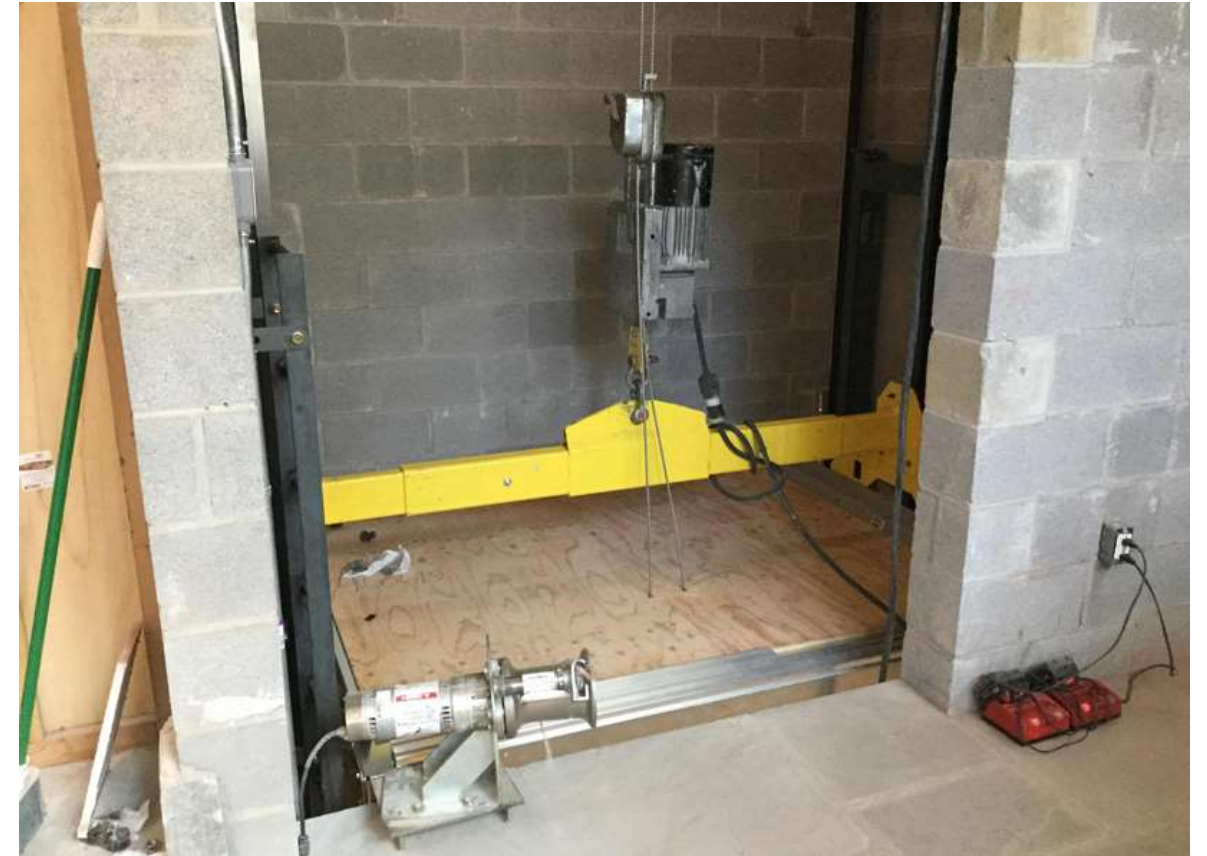
The two elevator installers make considerable progress.
