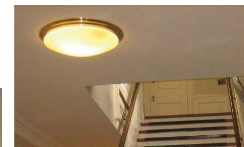
Light fixtures in first floor hall
