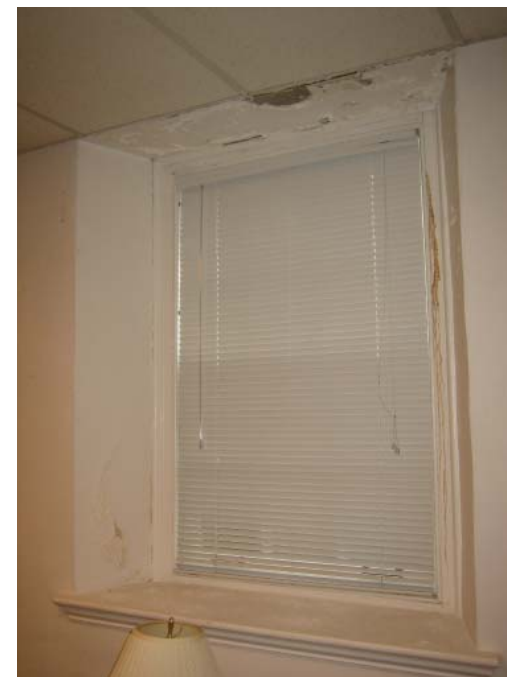
Window in Decatur Room (114)
