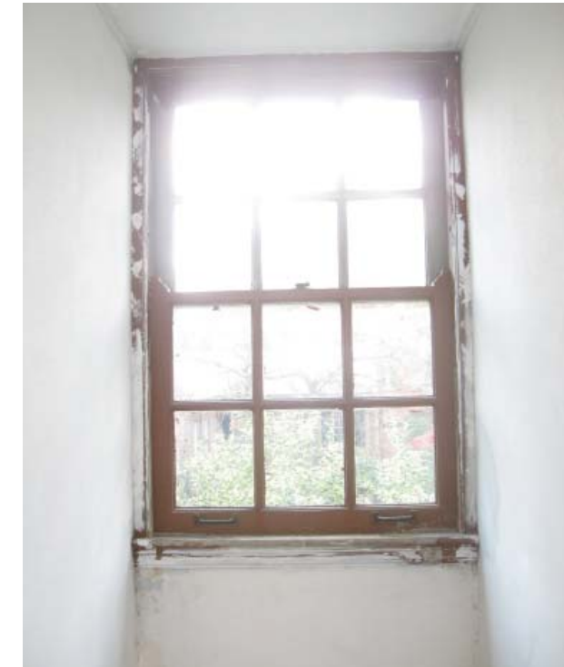
Dormer window at third floor in process of refinishing
