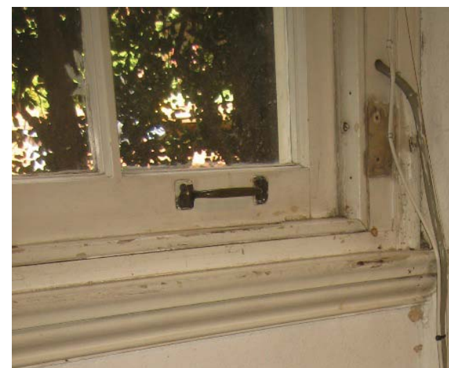
Window at office (108)
