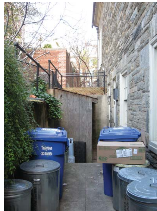
Areaway at kitchen where the new interceptor drains flow water to
