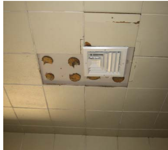
Acoustic tiles at classroom (204)
