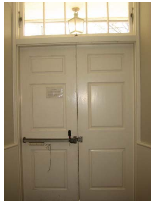
Second floor vestibule doors in hall
