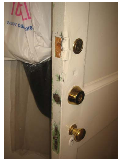
Door at office (112)
