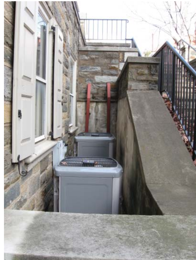
Areaways outside the Decatur Room with two red scuppers
