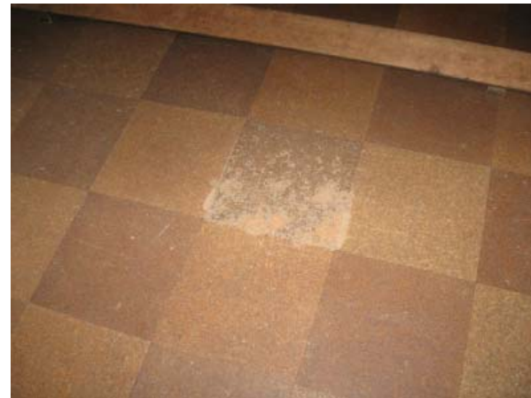
Cork tile flooring at Meeting Room
