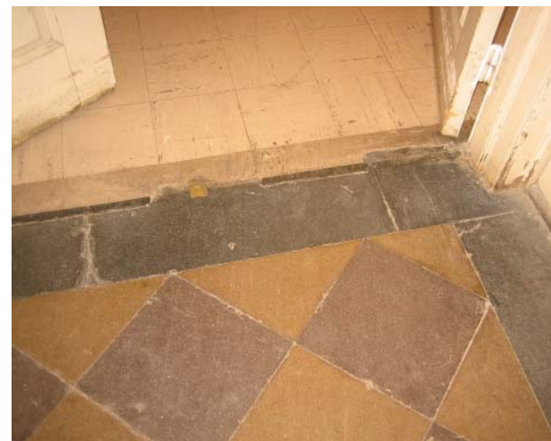
Original tile at storage room (102)
