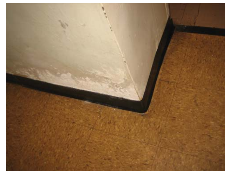
First floor hallway across from bathroom entrances
