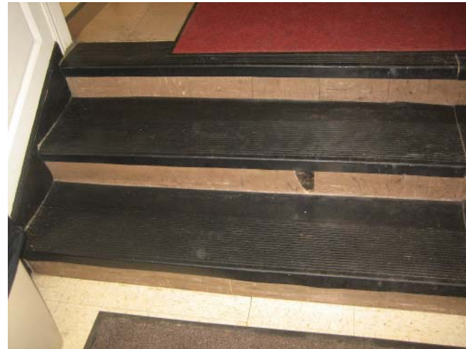
Entry vestibule stairs
