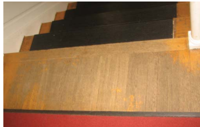
Wood flooring at second floor hall (207)
