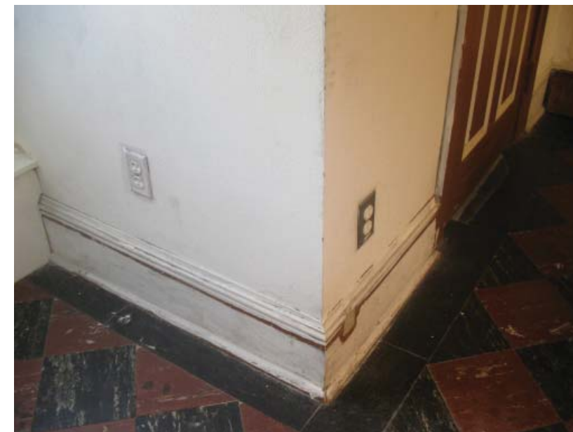
Baseboard and flooring at third floor hall
